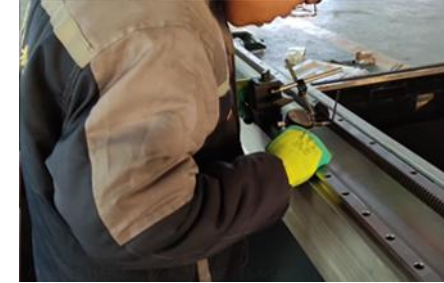
Rack installation and texting
