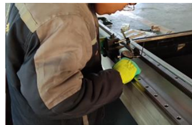
Rack installation and texting
